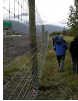
Wildlife exclusion fencing along the Trans-Canada Highway near Calgary, Alberta, Canada
